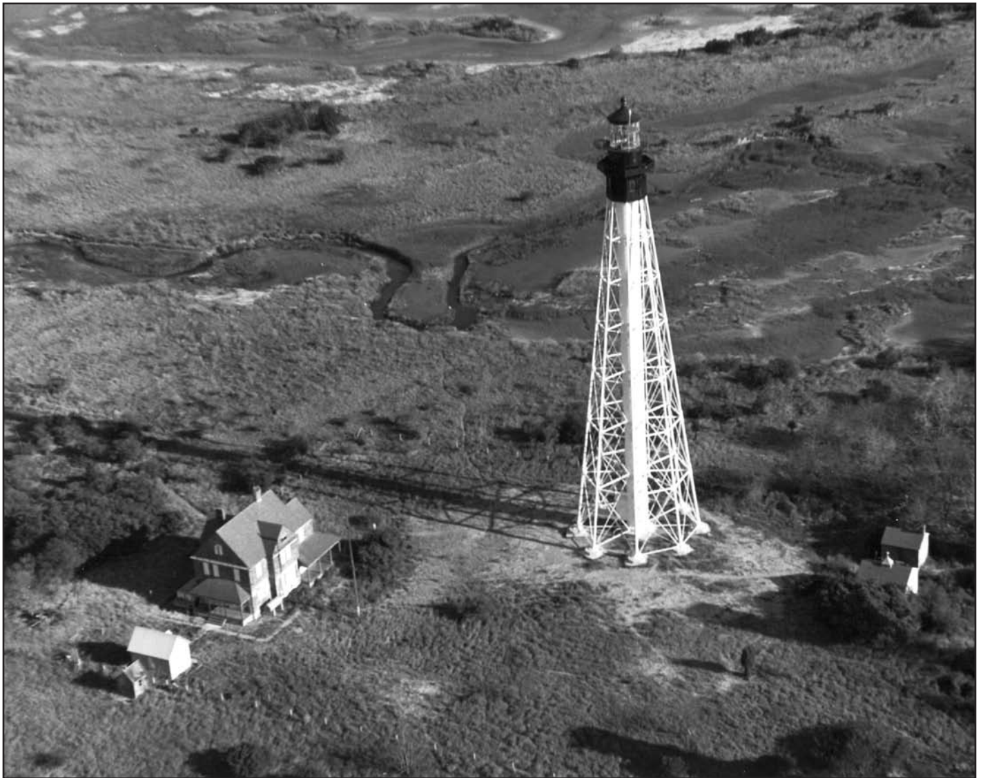
The Cape Charles Light Station in 1985. Duplex dwelling and store house at left, oil house and privy at right. Official U. S. Coast Guard photo by Kathi Bostman.
