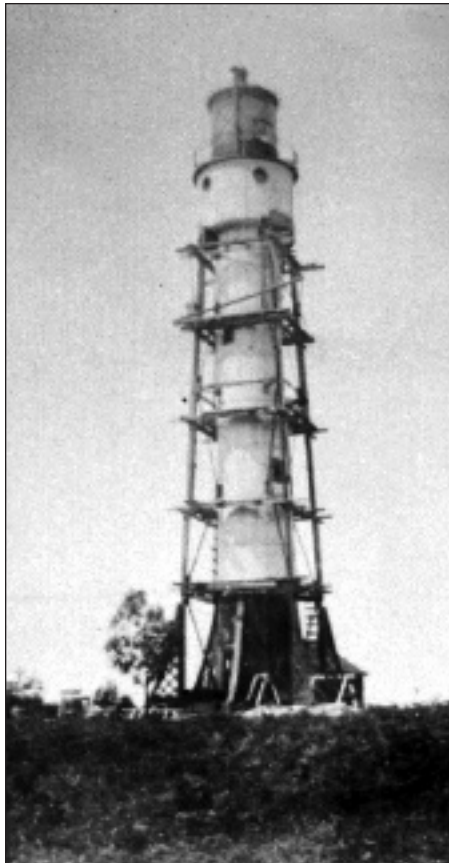
Left – 1914 view of the buttresses and support iron work at the foot of the tower to eliminate a vibration problem during high winds. Photo courtesy of Minnesota State Historical Society collection. Right – A more detailed view of the Devils Island iron and steel tower, showing the bracing which was added in 1914 to the unsupported structure. Photo courtesy of the author.
