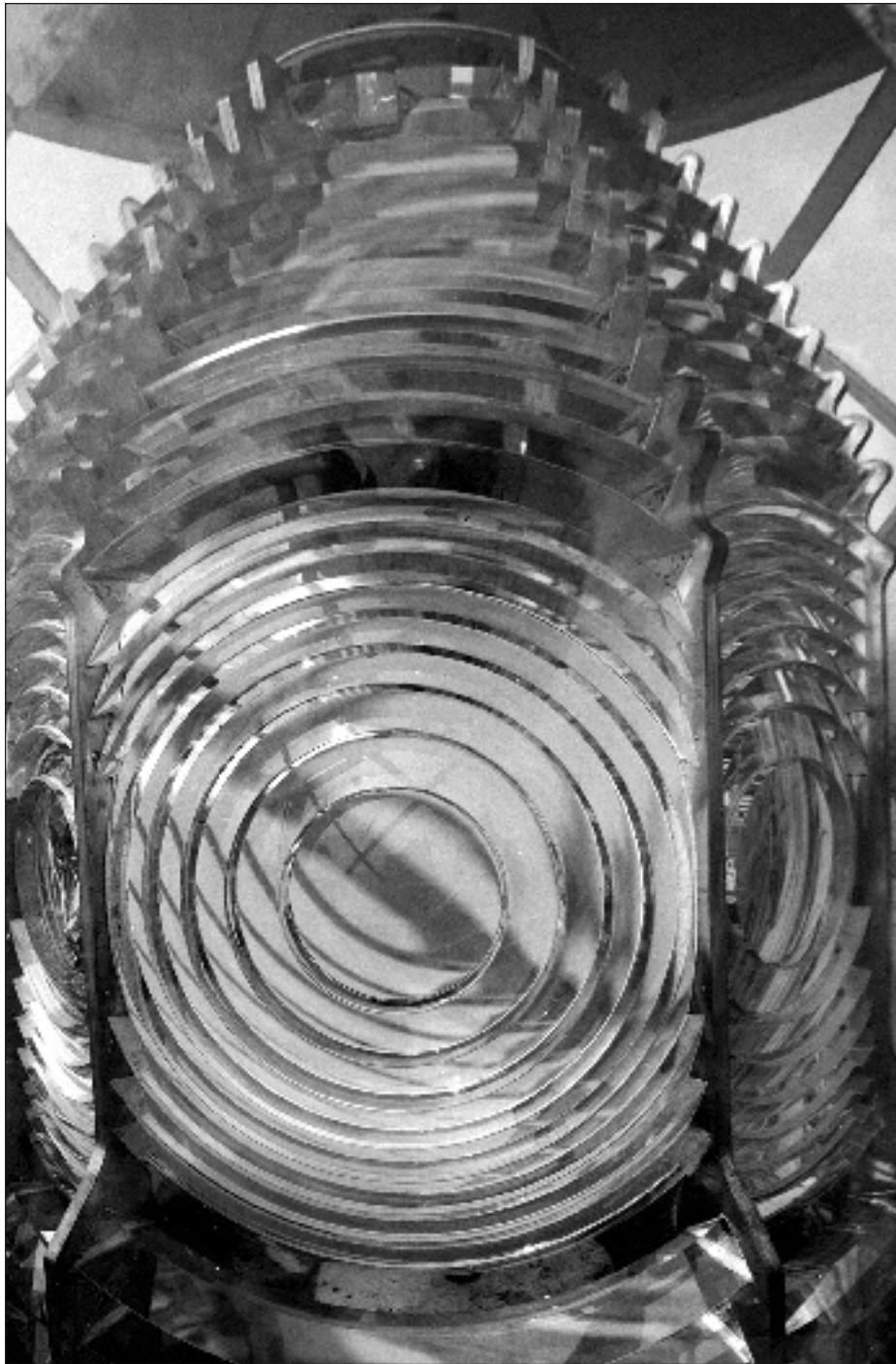
Above – An NPS employee working on the re-installation of the Third Order Fresnel lens in the Devils Island lantern, spring of 1976, photo by a local outfitter. Left – The Devils Island Third Order Fresnel lens in 2002. Photo by the author.
