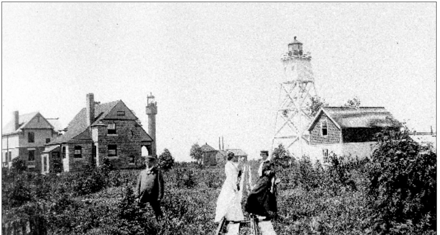
This fascinating photograph shows both the 1891 timber tower at right (behind the storage building) and the 1901 cast-iron and steel tower, left behind the dwelling. Note the absence of the structural bracing added in 1914. An oil house and fog signal building can be seen behind the ladies. They are standing on the tramway that runs from the landing to the fog signal building. U.S. Lighthouse Society photo.
