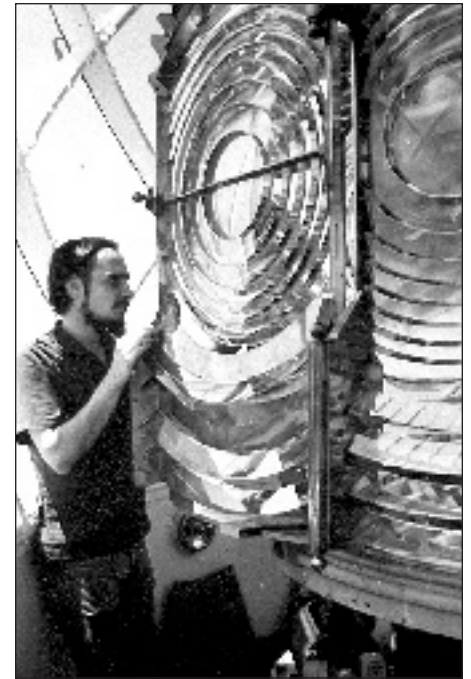
Above – An NPS employee working on the re-installation of the Third Order Fresnel lens in the Devils Island lantern, spring of 1976, photo by a local outfitter. Left – The Devils Island Third Order Fresnel lens in 2002. Photo by the author.
