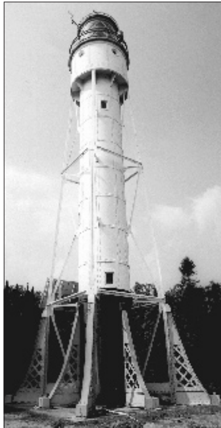
Left – 1914 view of the buttresses and support iron work at the foot of the tower to eliminate a vibration problem during high winds. Photo courtesy of Minnesota State Historical Society collection. Right – A more detailed view of the Devils Island iron and steel tower, showing the bracing which was added in 1914 to the unsupported structure. Photo courtesy of the author.
