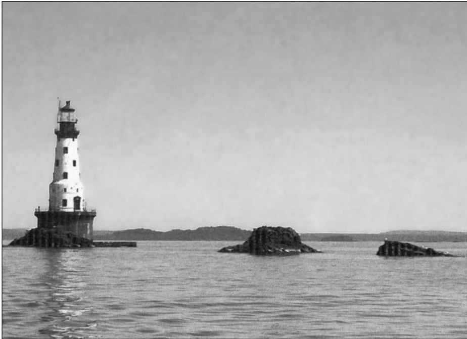
The reef off of the Rock of Ages which the vessel George M. Cox struck. Note the lens has been removed from the lantern room. 2002 photo courtesy of Darrell Camp.
