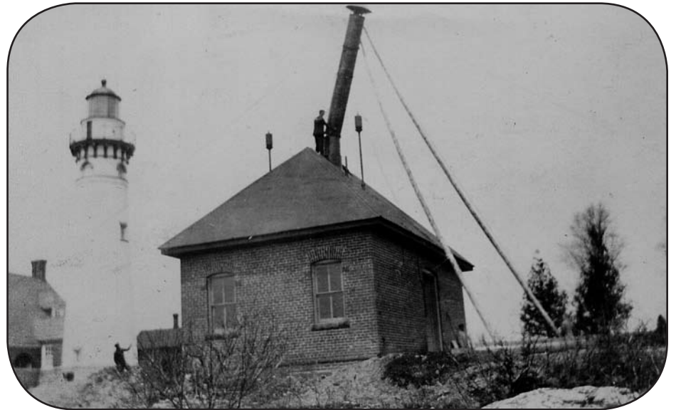
Above – Working on the chimney of the Seul Choix fog signal building. Note the two whistle fog signals on either side of the chimney. Photo courtesy of the author. Below – Workers install a boiler for a steam-powered fog signal. Lighthouse Society photo.
