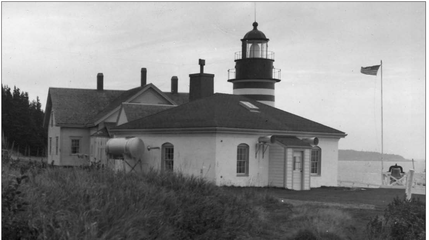
Above – Fog signal house showing the dual fog trumpets. Note oil tank at left for fueling the boiler and at far right, the fog bell. Photographer unknown.
