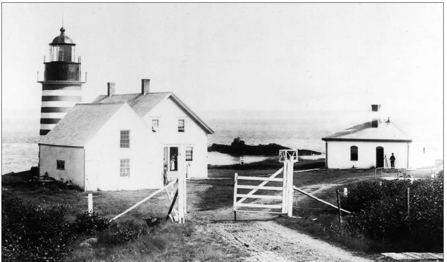
Below – View of the light station circa 1880s. Note the keeper in front of the fog signal building and keeper's wife in doorway of dwelling. Photographer unknown.
